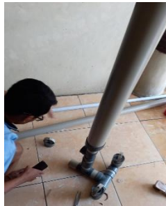
Figure 3. Hidram Pump Assembly 2 katup buang PVC 2"
