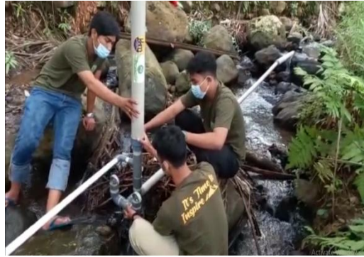
Figure 8. Installation of Hidram Pumps in selected Areas
